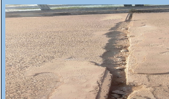
Picture 2.18: Absence of expansion joints in bridge across Swarnrekha river between Khokro-Karkidih road in Ichagarh block of Saraikela district
