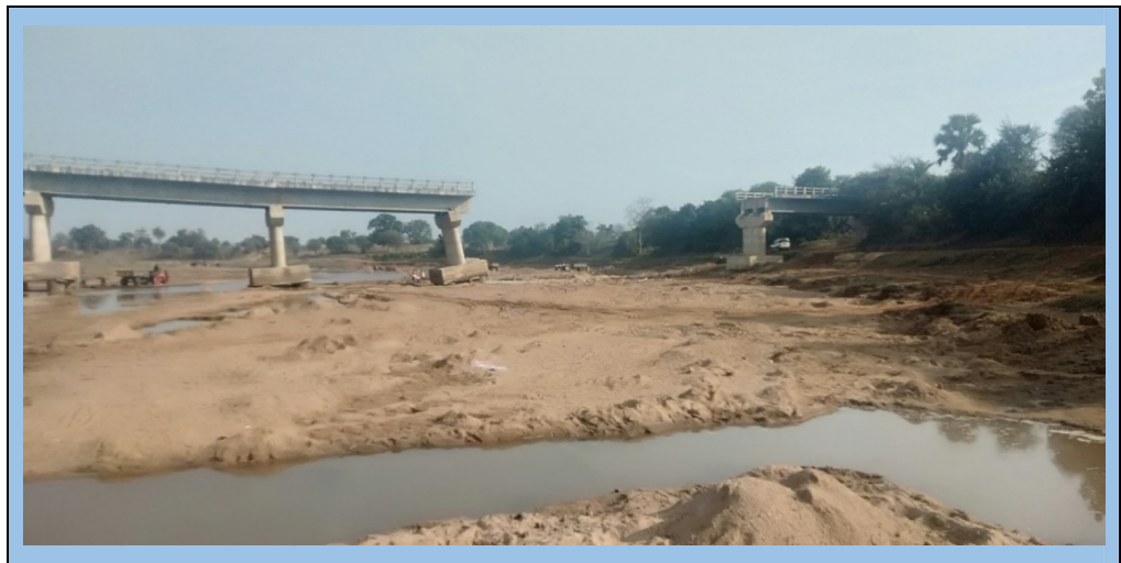
Picture 2.13: Damaged spans of bridge over Bansloi river in Chandalmara in Pakur district
