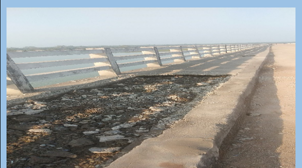
Picture 2.19: Broken slab in footpath in bridge across Swarnrekha river between Khokro-Karkidih road in Ichagarh block of Saraikela district
