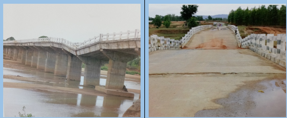
Picture 2.10: Photograph of damaged bridge over Sankh river between Mariyam toli-Sarnatoli in Raidih block
