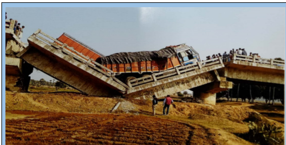
Picture 2.14: Damaged span of bridge over Korka to Pakaria road in Pathargama block of Godda district (Photo taken from files of the division)
